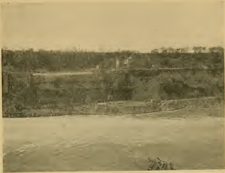
SITE OF THE POWER-HOUSE OF THE ONTARIO POWER COMPANY AT THE EDGE OF THE WATER BELOW THE FALLS ON THE CANADIAN SIDE.
